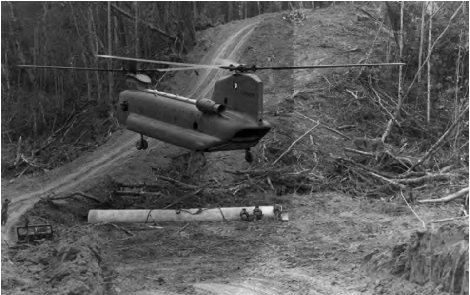
A CH-47 Chinook helicopter drops off preassembled culvert on Route 547.
